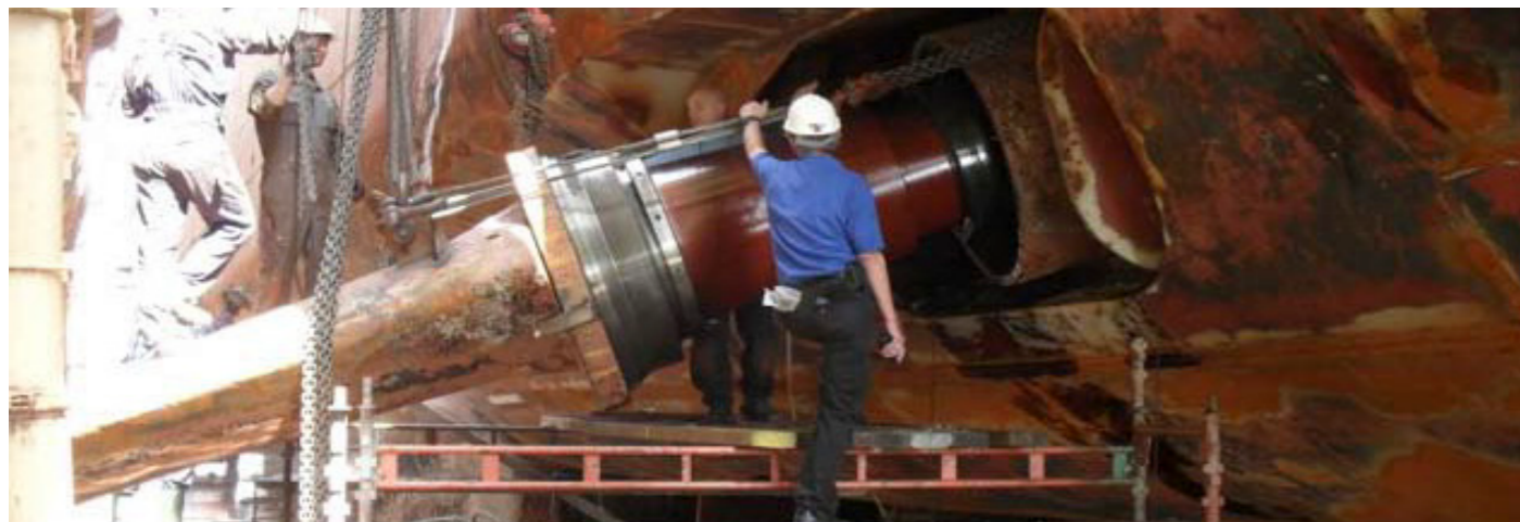
Removal of fin and shaft (for shaft seal replacement)
